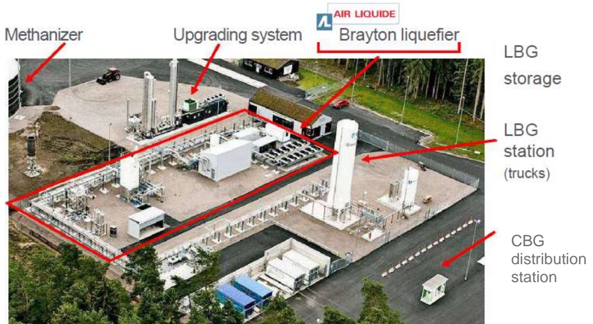
Figure 4. Air Liquide biomethane liquefaction plant (13 TPD) in Lidköping, Sweden [Air Liquide 2013].
